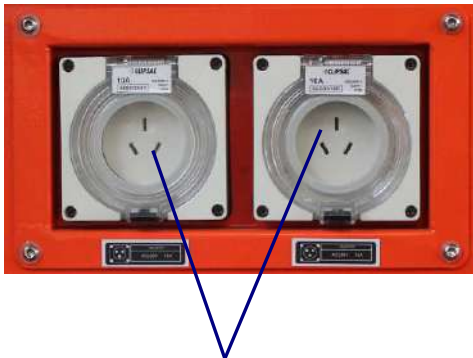
Standard power socket outlet (10A, 1Phase, 220V)
